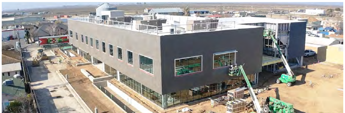
Bush Construction: Firebaugh Center, West Hills Community College District
